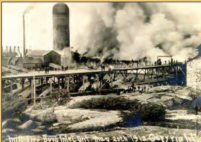
The Graves Bigwood sawmill was built and completed by 1902 and eventually became the largest mill of its kind in Canada. The mill and its facilities covered over one square mile of land consisting of: a large lumber yard, green lumber yard, planing mill, 11 wood-fired boilers for steam power, dock slips and a box factory. In the spring of 1912 the original mill burnt down. It was rebuilt that fall.
