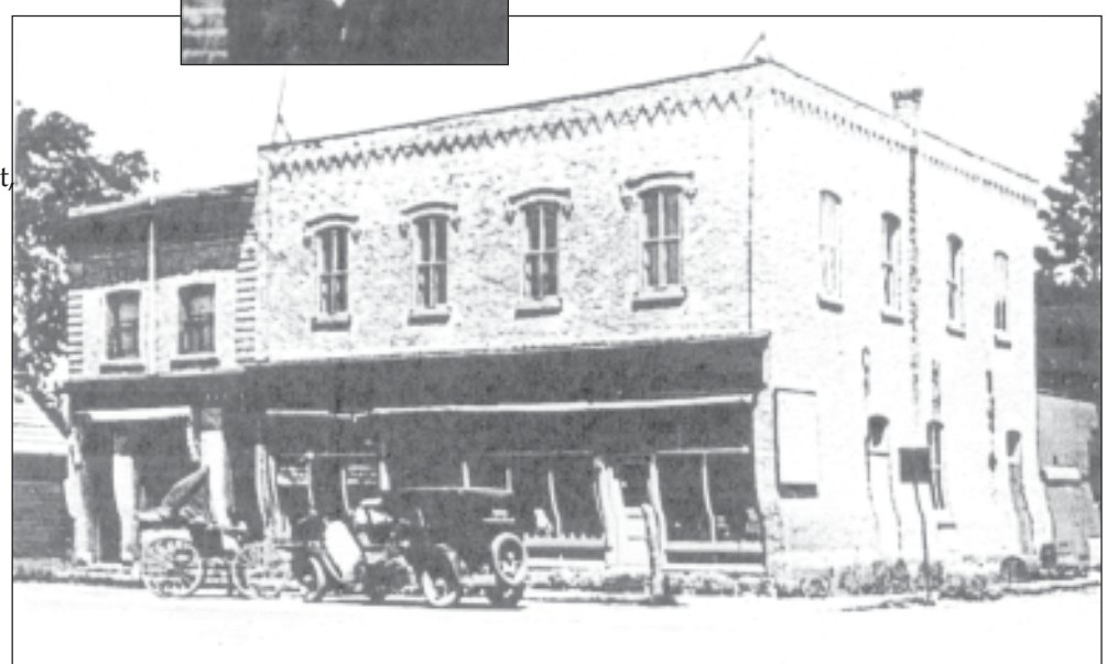
The Rourke, Lyne & Atchison General Store. William F. Brown, postmaster from 1936 until 1944, operated from a room at the front right of the building which was home to the post office during his tenure.
