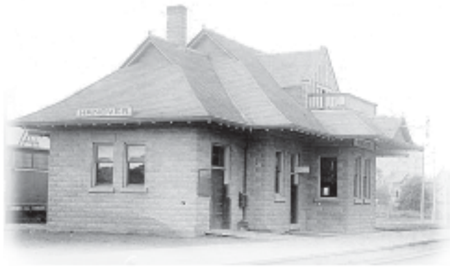
Grand Trunk Station (CNR), Hanover, Ontario.
