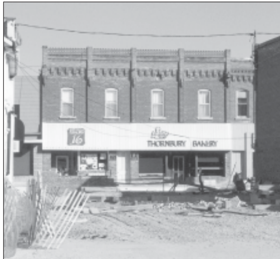
For the moment all that was left was but a hole where the post office had stood for the past 45 years. Even that reminder was gone within the week in preparation for the creation of a small parkette joining Bruce St. to the Hester St. parking lot.
