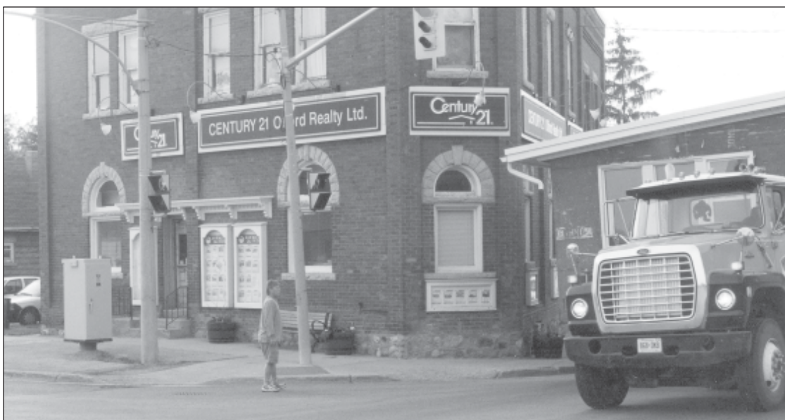
6:17 a.m. and the post office is slowly moving west through the intersection passing the old Bank of Toronto building, now a real estate office. The building has not altered much in appearance since 1907. The front entrance has been removed and the old entrance to the post office is now the entry into the real estate office – just to the right of the light standard.
