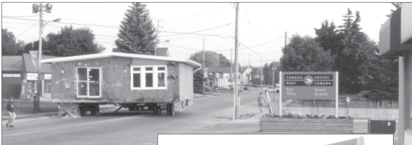
6:20 a.m. – The move is almost completed as the building is about to turn right onto the vacant lot just beyond the Canada Post sign. The move was completed at 6:24 a.m. Getting the post ready took a couple of weeks; moving it took just a few minutes.
