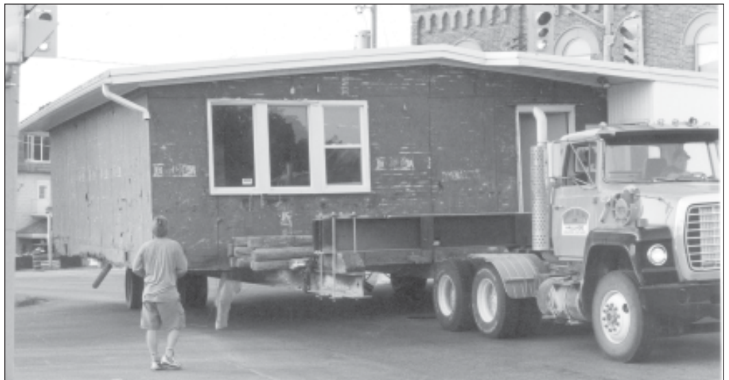
6:15 a.m. and the post office building is slowly moving into the intersection of Bruce and Bridge Sts. We are looking the back of the building where the mail truck would have its daily pick-up and drop-off.
