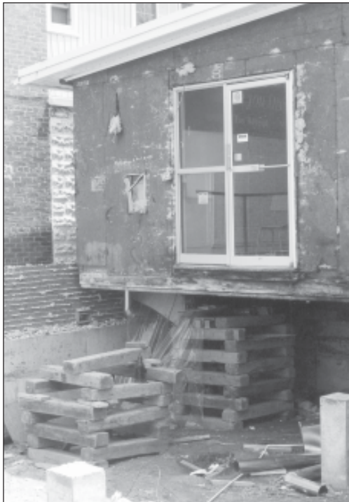
The post office is being prepared for the move by first having its brick veneer removed and then jacking up the building in preparation for the beams and moving wheels. Notice the mail drop to the left of the front entry.
