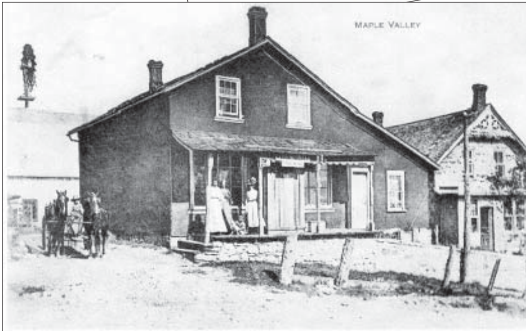
The post office at the home and store of W. D. Taylor. In 1884 Mr. Taylor had purchased the store property from Henry White and commenced a business of servicing pumps and windmills, as well as digging wells. He became postmaster in 1899.
