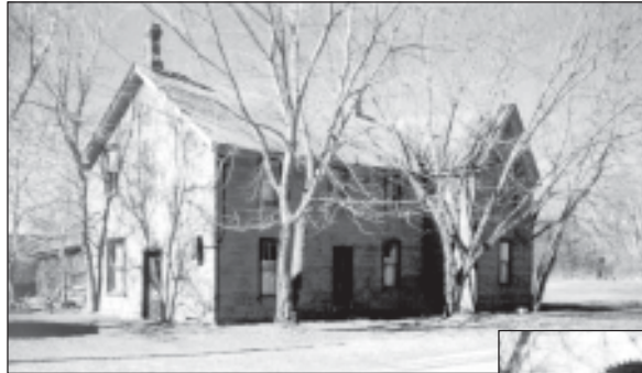
The Rock Mills post office as it appears today in the winter of 2000.
