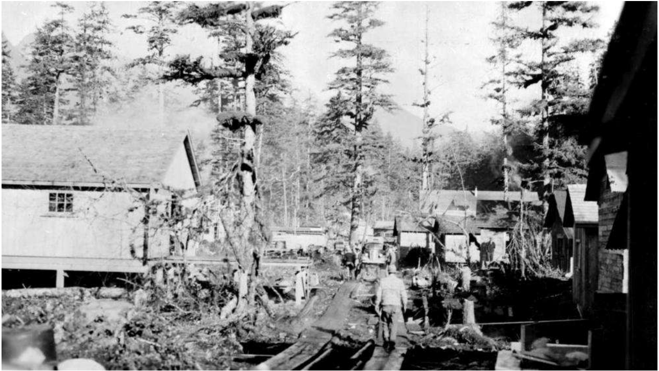
Figure 23. Board road at the lower end of the Zeballos townsite (February 1938). BC Archives Item G-02459
