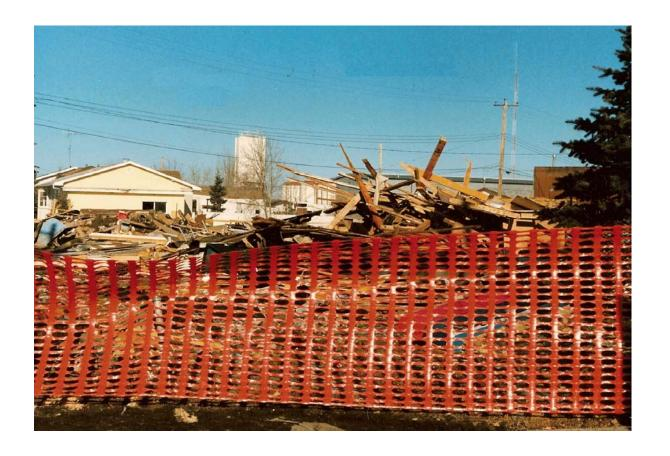
On 1990-03-02, a Friday, the Blackfalds post office was c o m p l e t e l y obliterated by a natural gas explosion. A main line in the street had been leaking at a union, and the gas flowed sideways underground into the post office basement [5].
