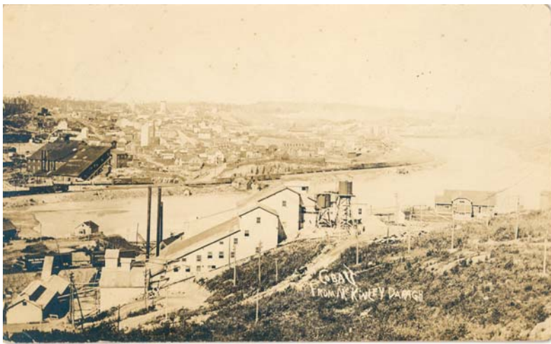
Fig. 5 – A postcard view of Cobalt and the McKinley-Darrogh mine, showing mine head-frames, waste tips and the ore reduction stamping mill (the dark building on the left). The message on this postcard, carrying a 1913, North Bay & Cochrane RPO, was “This gives a good idea of what a silver mining camp looks like”.
